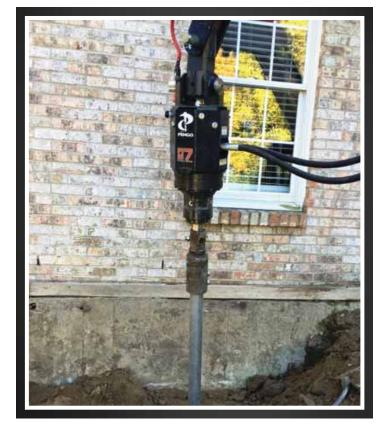
Choose the single speed RS-7 anchor drive for your next installation project. The standard cross-over pressure relief system will protect the hydraulic motor from pressure spikes and potential overload conditions. Add a mount and the TruLink® for the complete drive system.
